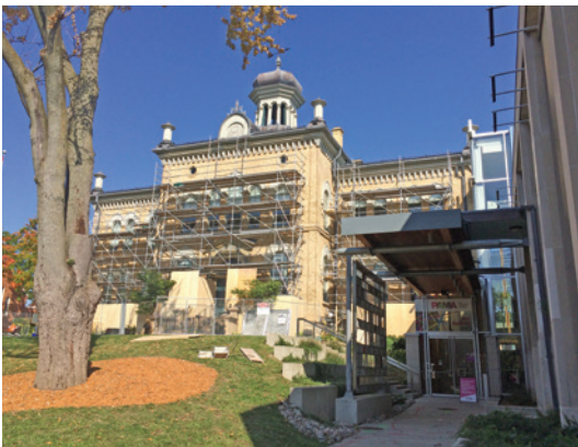
Hoarding on the front of the courthouse allowed for the repair and refurbishing of the wooden sash windows .
